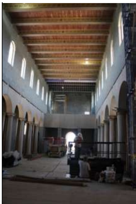
(Ceiling and columns in FSSP new seminary chapel, NE)
